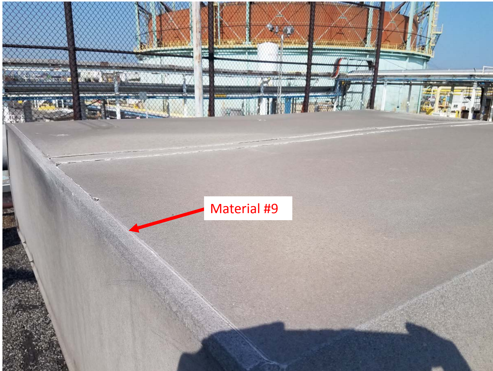
Photo 4: Norwest Building white caulk on air intake ductwork (Material #9).
