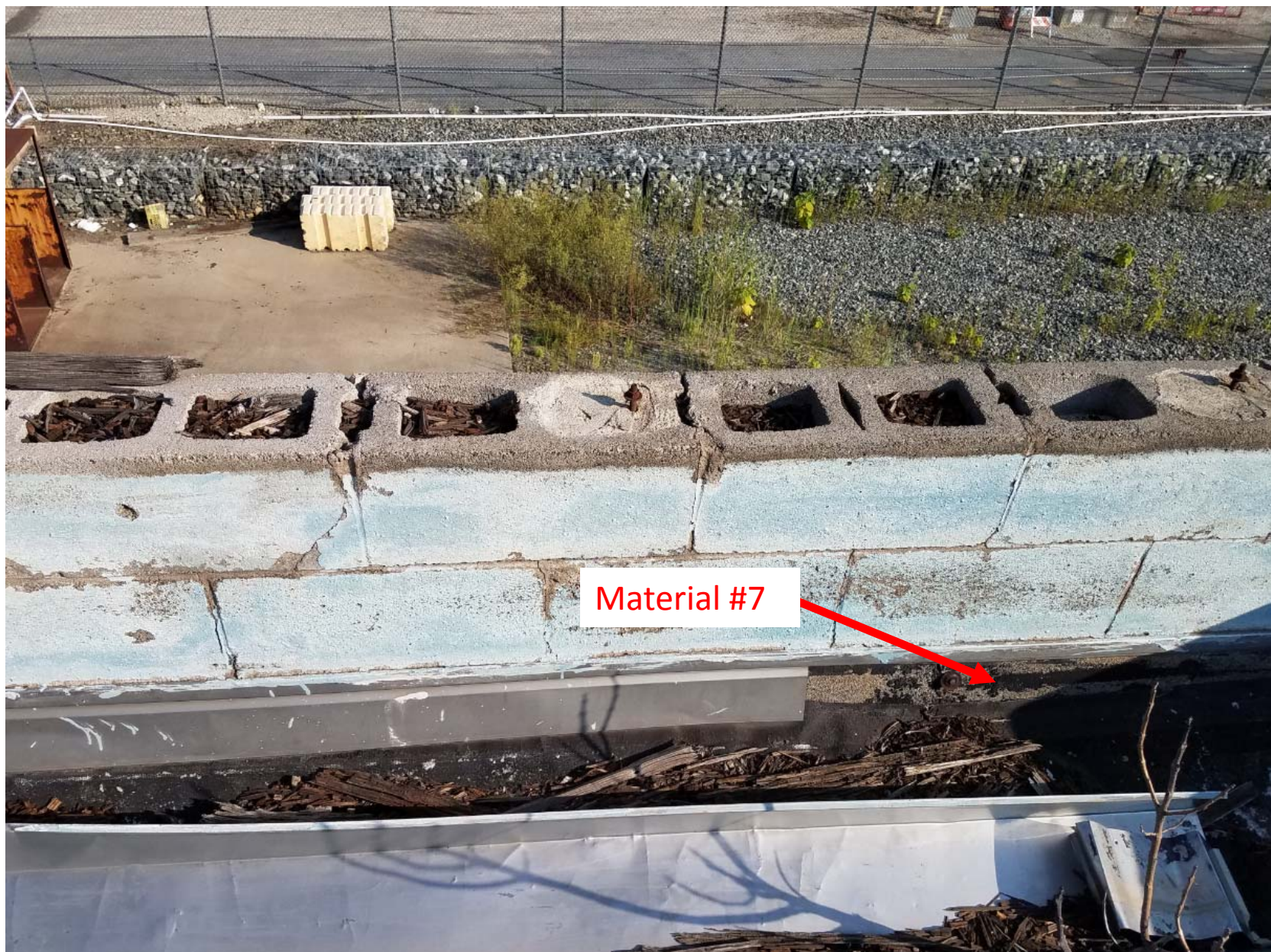
Photo 3: Northwest Building gray-black roofing cement (Material #7).
