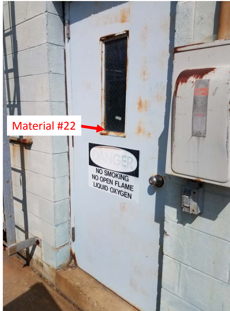
Photo 7: Northwest Building exterior door at south wall. Window glazing is ACM (Material #22).
