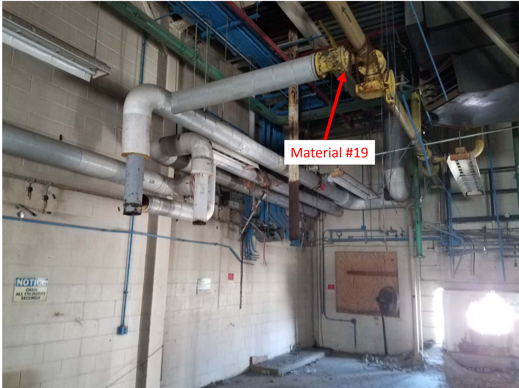
Photo 6: Northwest Building interior. Gaskets (Material #19) on all piping are ACM.
