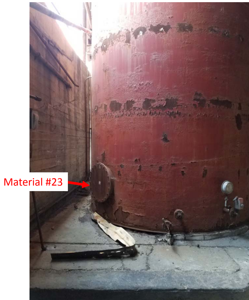
Photo 9: Asbestos-containing gaskets (Material #23) on red tank in NW corner of Main Building. Gaskets also observed on top of tank.
