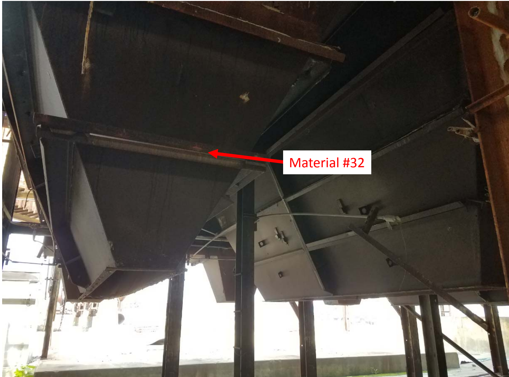
Photo 10: Asbestos-containing gaskets on baghouse adjacent to Main Building (Material #32).
