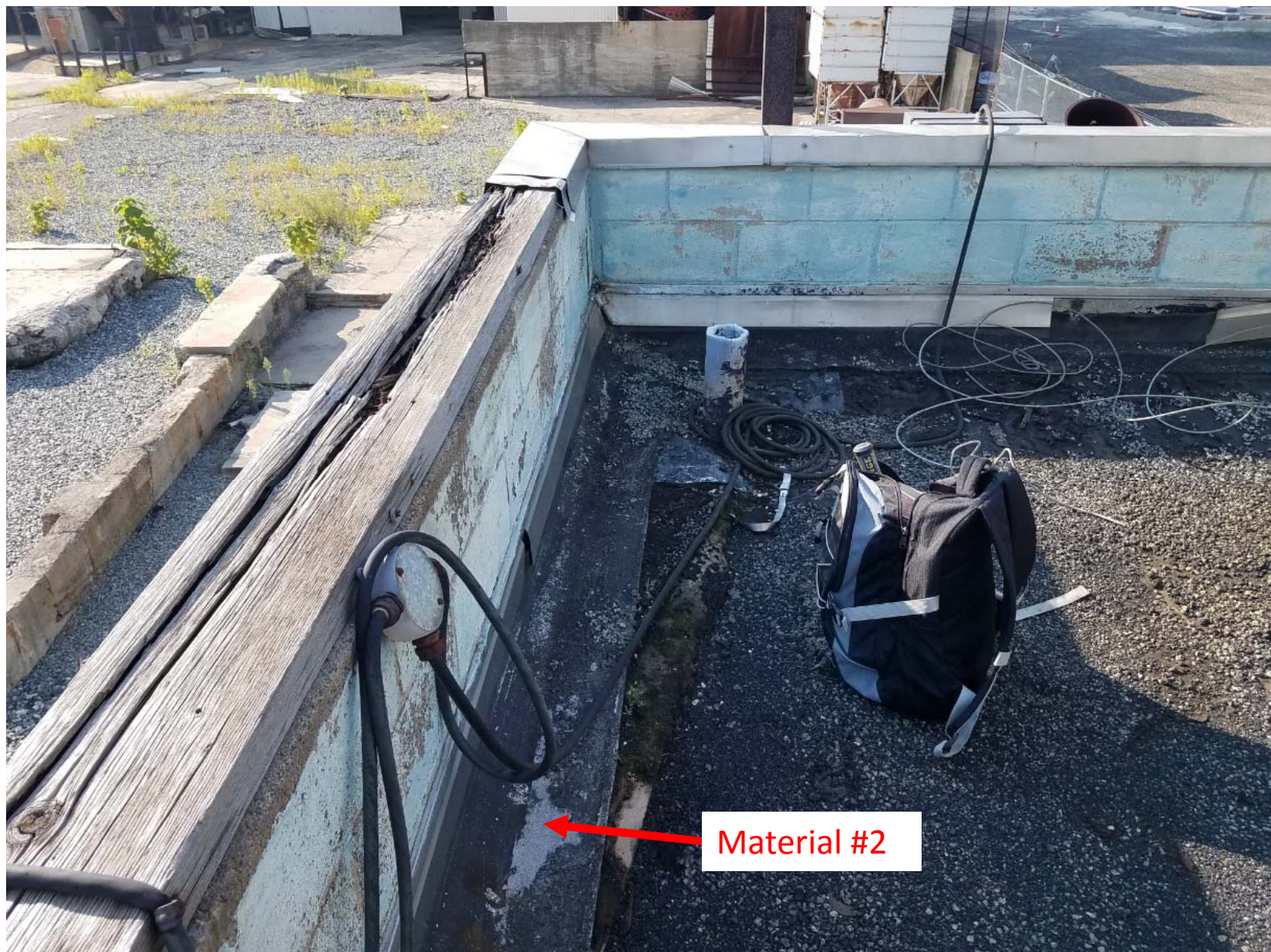
Photo 2: Northwest Building perimeter roof flashing close-up (Material #2).
